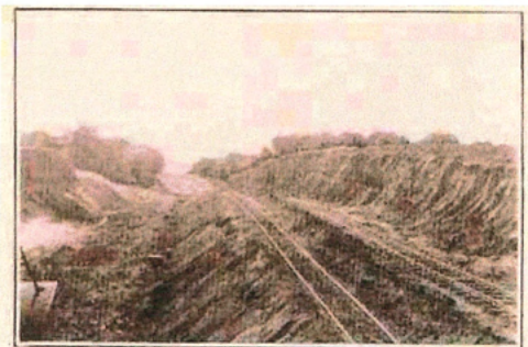
Temporary Track Used to Transport Filling Material
