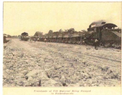
Thousands of Fill Material Being Dumped in Embankments
